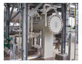
LiquiSep®protects critical assets from water contamination and the salts, acids and bases which it may contain. The application of LiquiSep®allows optimized performance of downstream treaters, salt beds, exchangers and reactors while assuring the elimination of haze from finished products.
